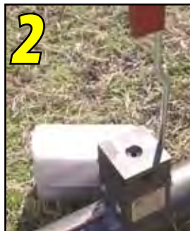
2 Position conductor and mold onto pipe.
