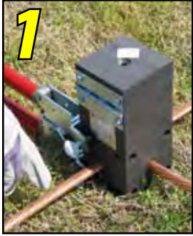
Position cleaned conductors in mold
