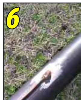
6 Remove and clean mold before making next connection.
