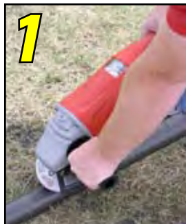
1 Clean pipe before making weld.
